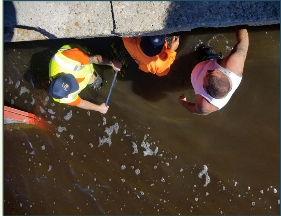
OF-0142 (After): completing valve installation
