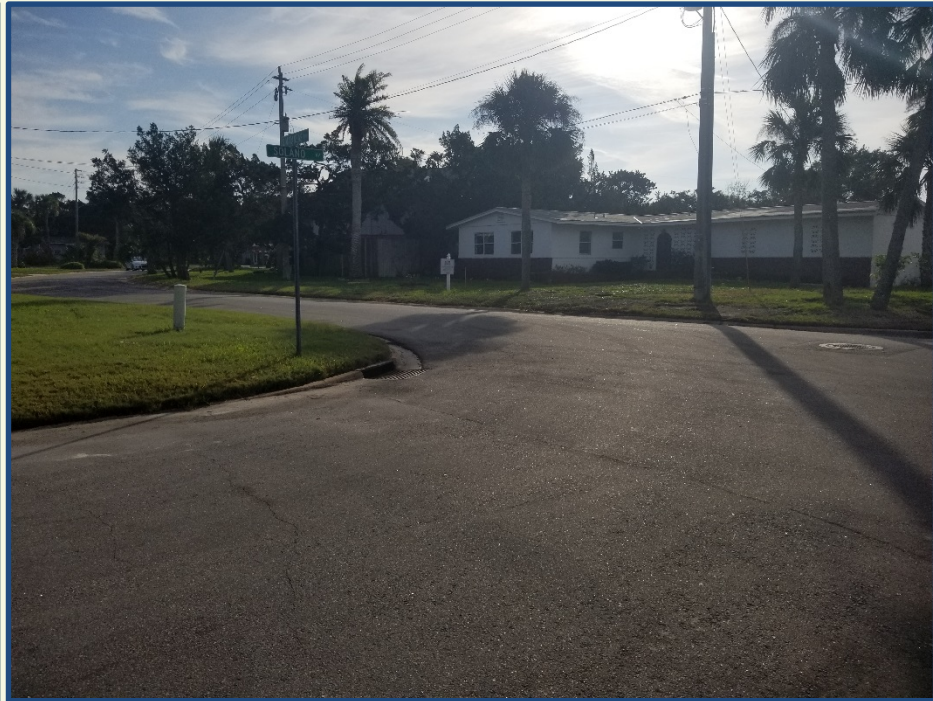
OF-0117 (After): no street flooding during King Tide event (December 2017) - tidal flooding eliminated
