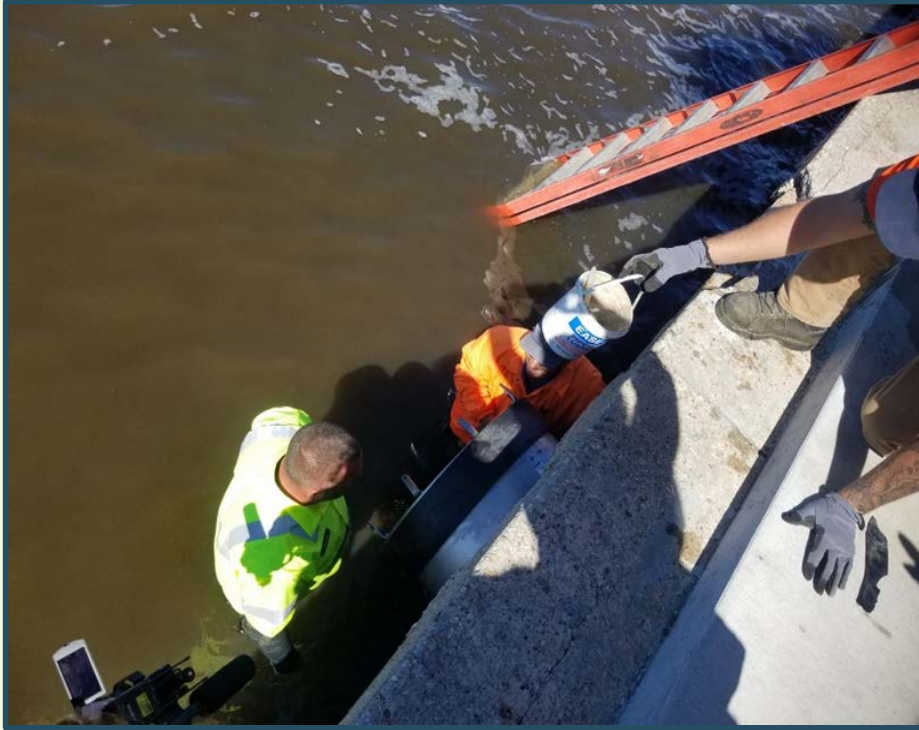
OF-0142 (After): valve inserted into outfall pipe
